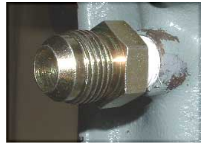
AN-12 Fitting installed in bypass hole Be careful when installing. Use Teflon tape and do not over tighten.
